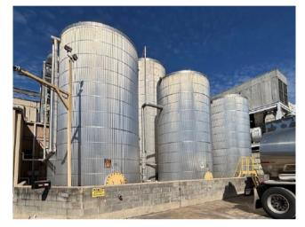
PVA Recovery at our Blacksburg, Textile Manufacturing plant (U.S.). PVA is recovered from wastewater and the water is reused for other textile operations.
