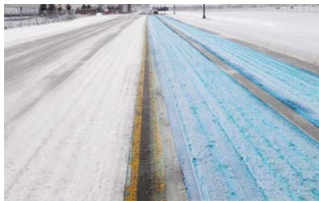
A comparison between traditional de-icing technology using the innovative Milliken Liquitint ® Winter Colorant applied by the Delaware Department of Transportation.
