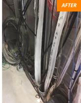
After the innerduct was extracted, the MaxCell team was able to install 4 packs of 3", 3-cell MaxCell fabric innerduct in each conduit structure. MaxCell was able to reclaim and provide 24 new pathways for future cable installation – where there was previously none. This allowed immediate deployment of new bandwidth while preserving space for future needs.
