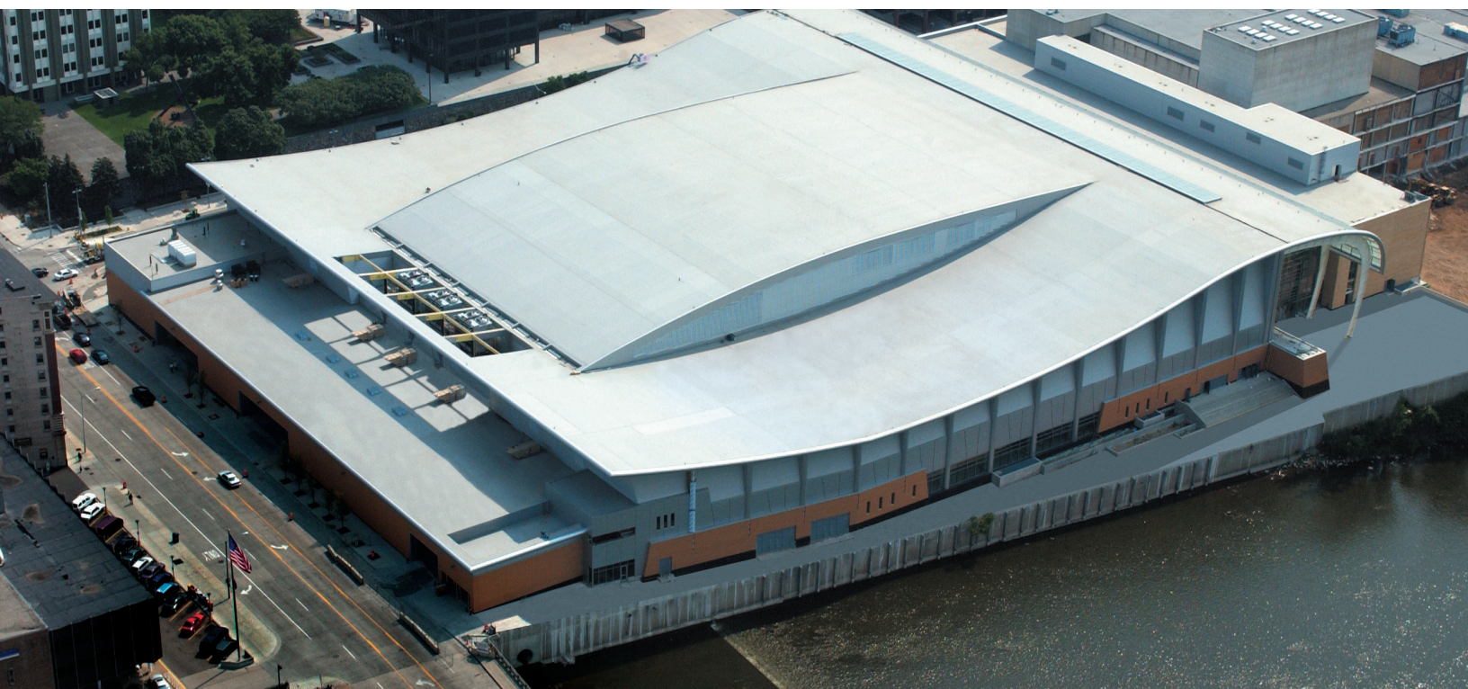
Single ply roof using a Milliken reinforcement.
